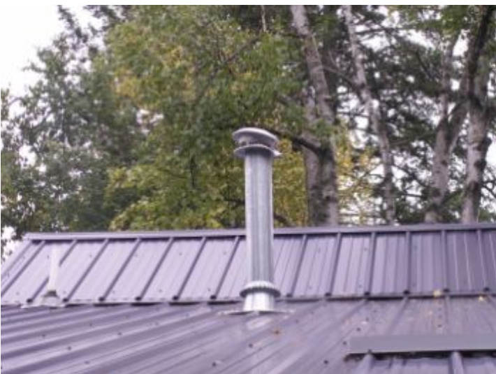
Furnace vent appears to have been hit with a tree branch. Cosmetic issue.
