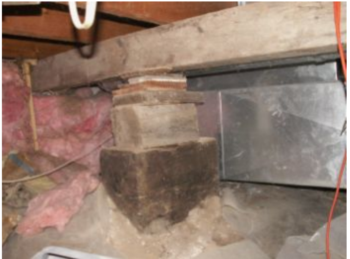
Crawlspace. Girders supported by stacks of wood blocks.
