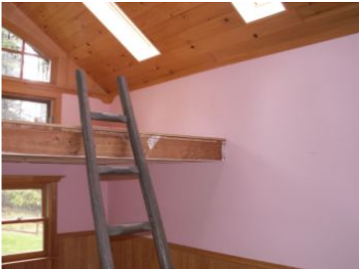
Interior of bunkhouse. No deficiencies observed.
