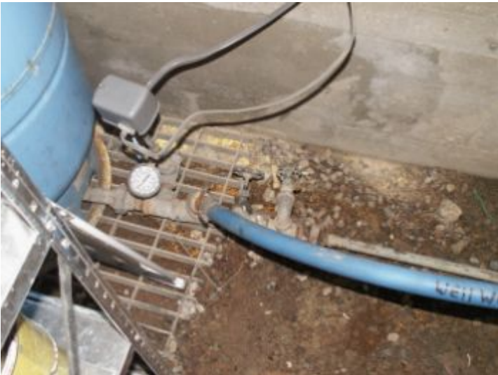
Water shut off for the house. No deficiencies observed.
