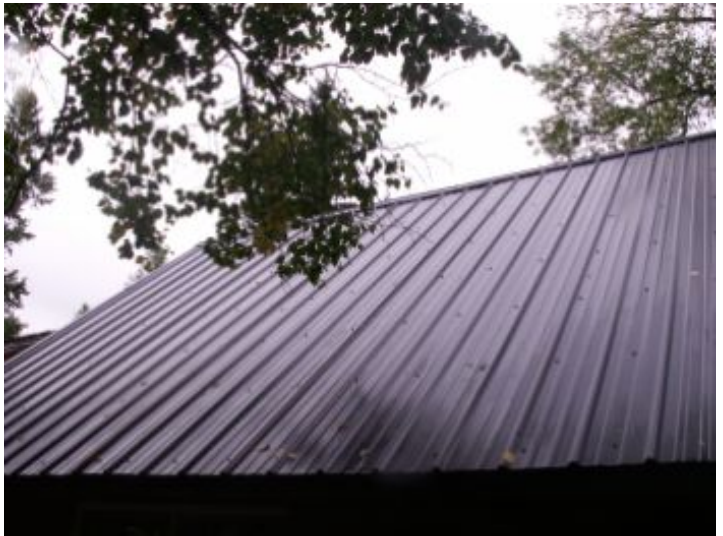
Metal roofing. No deficiencies observed.
