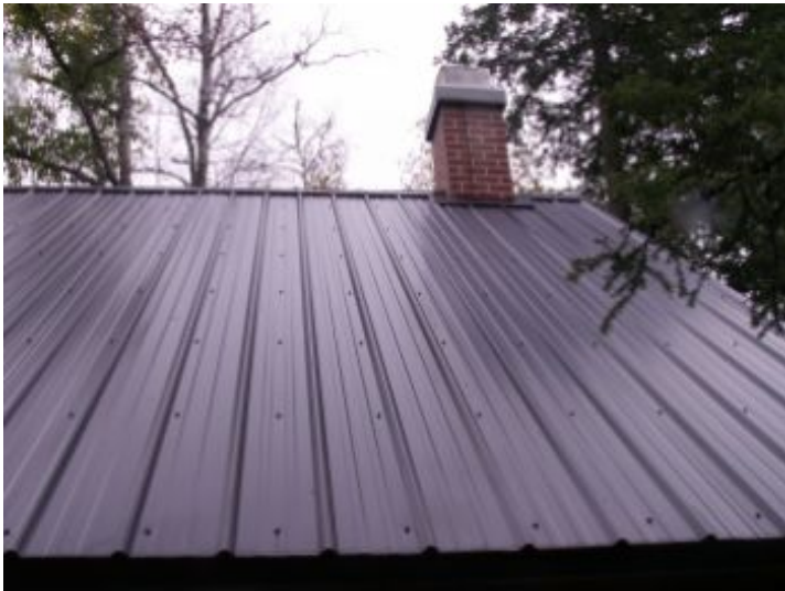
Old chimney not being used,
