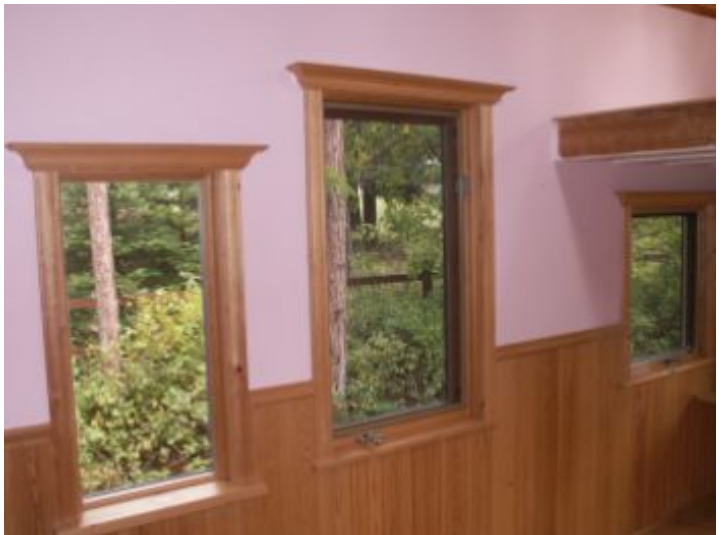
Interior of bunkhouse. No deficiencies observed.
