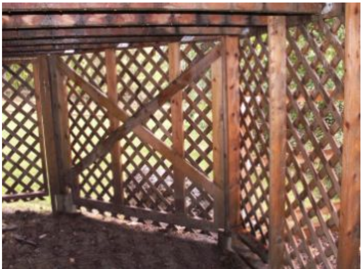
Deck framing. No deficiencies observed.
