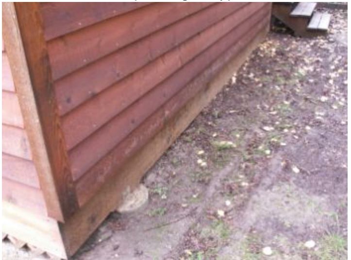
Bunkhouse supported on concrete piers. No deficiencies observed.
