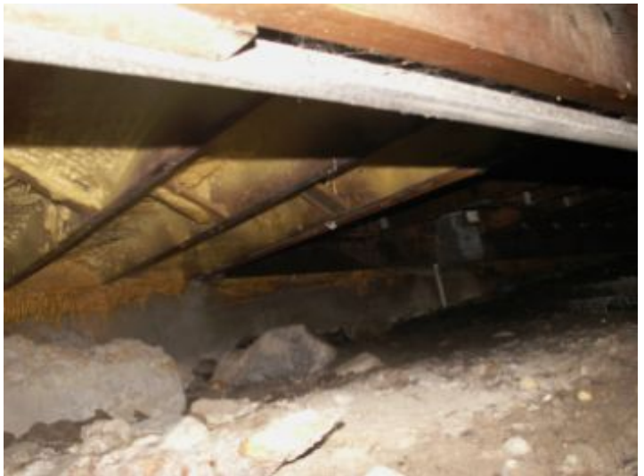
Spray foam insulation below dining room. No deficiencies observed.
